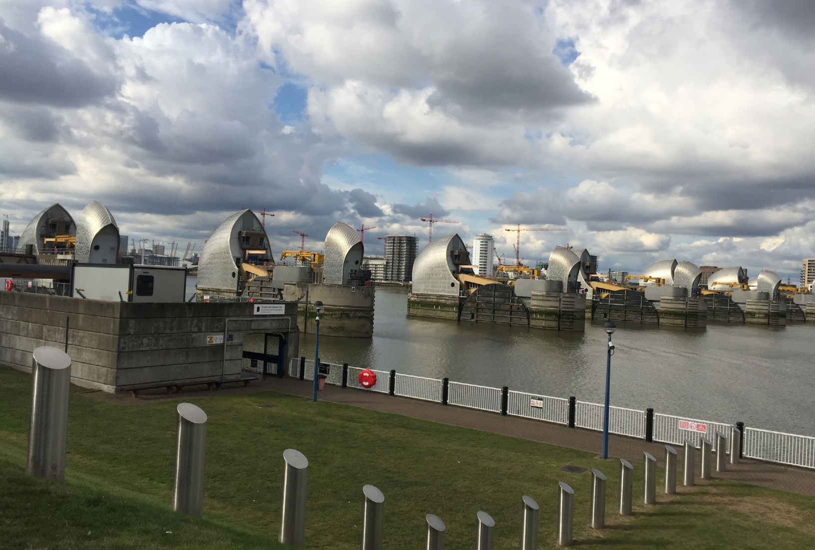
Thames barrier—London’s major flood protection against storm surges and high tides. Photo credit: Salem Afeworki.
