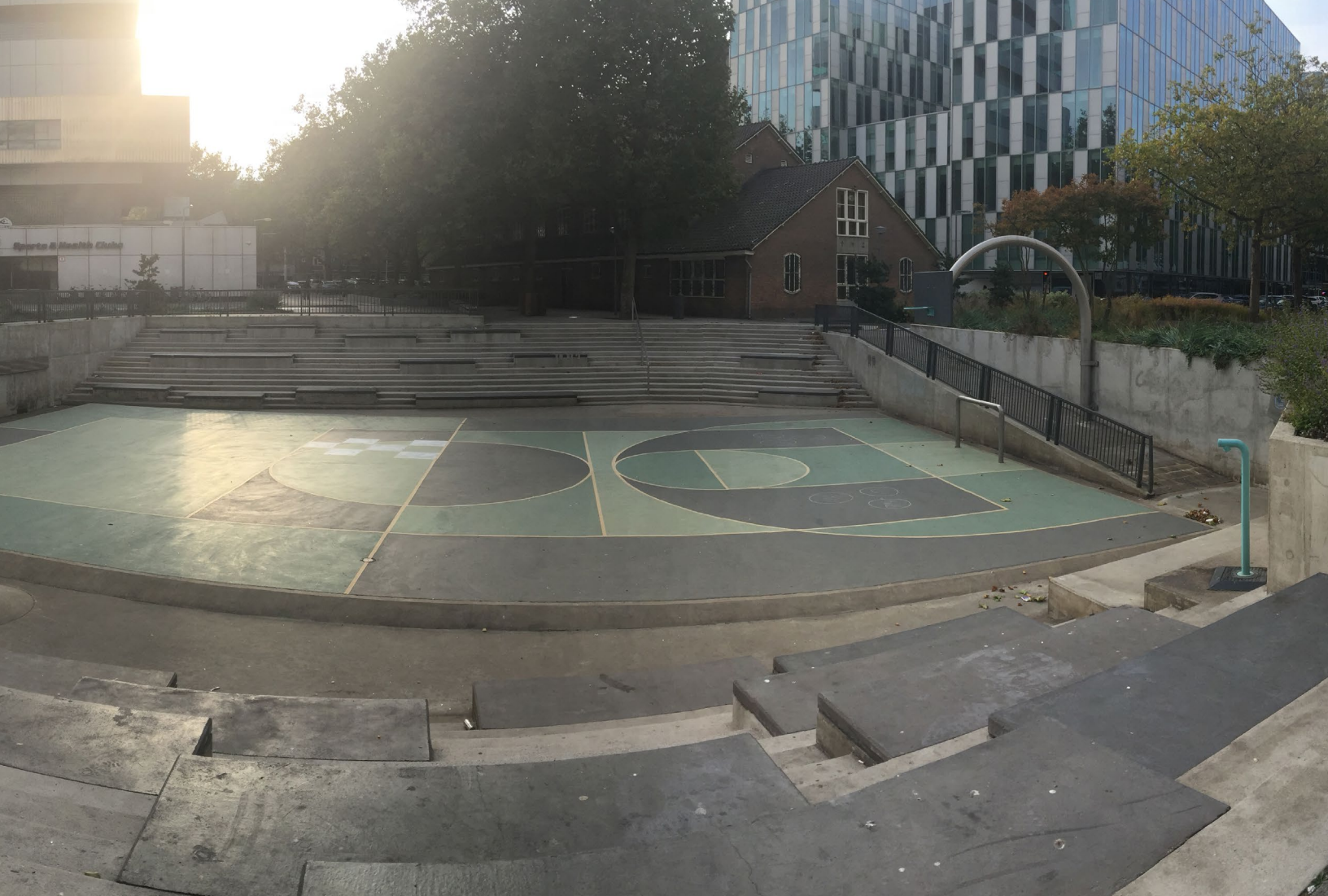
Watersquare Bethemplein in Rotterdam—the world first combined water retention and public square designed by De Urbanisten. Photo credit: Kate Judson.
